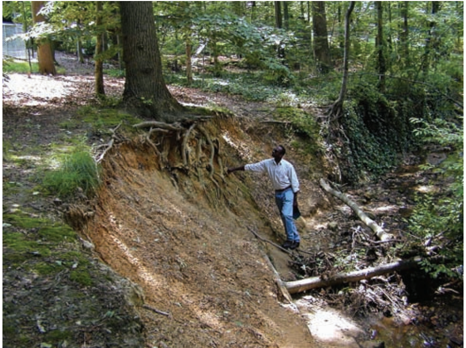
Eroded stream banks caused by excess stormwater runoff.
